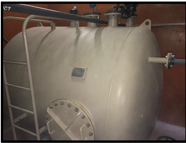
20m 3 steel vacuum tank
