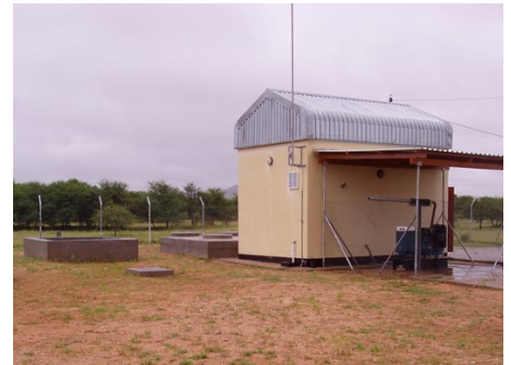
1 of 2 Vacuum Stations with Biofilter and Genset (front)
